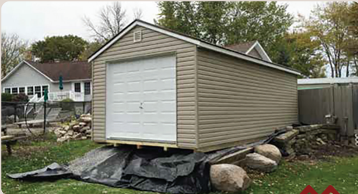
SHED DELIVERED ON UNPREPARED SITE
