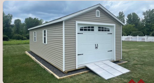
STRUCTURE DELIVERED & PLACED ON PROFESSIONAL STONE PAD
